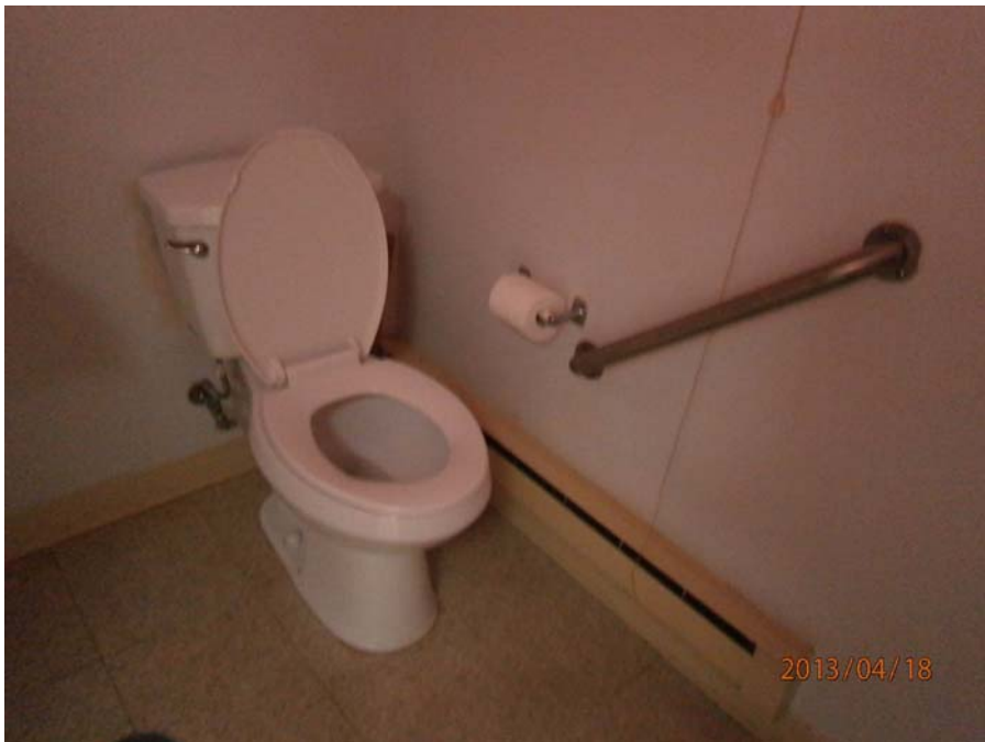
11. Common area restroom - note grab bars
