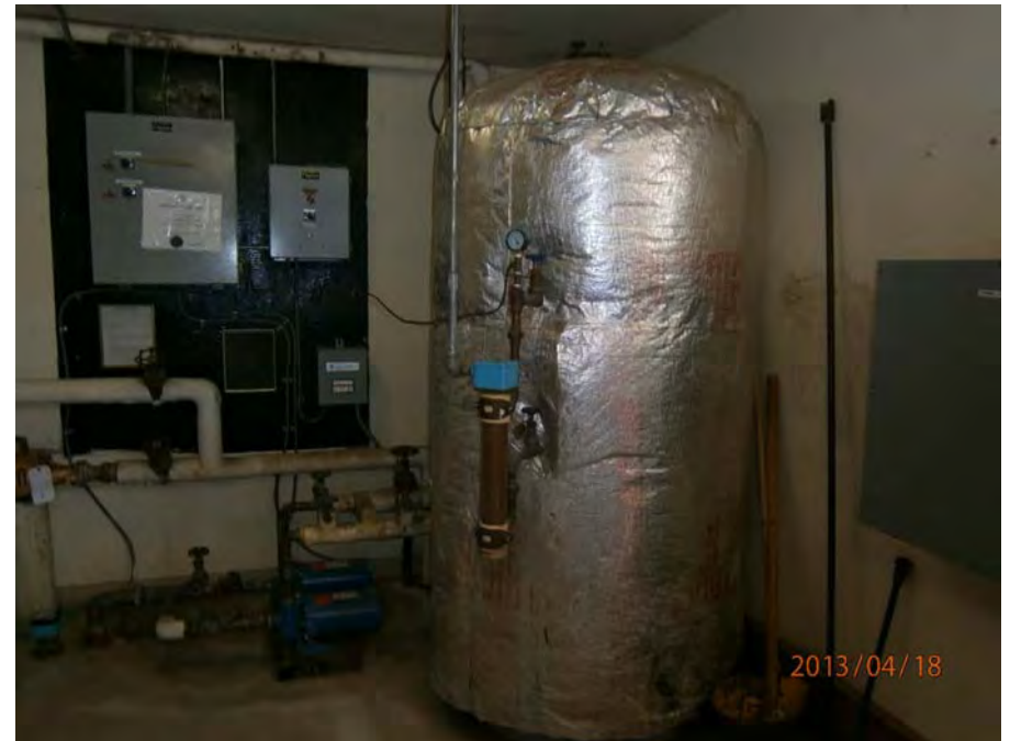
14. Well water storage tank
