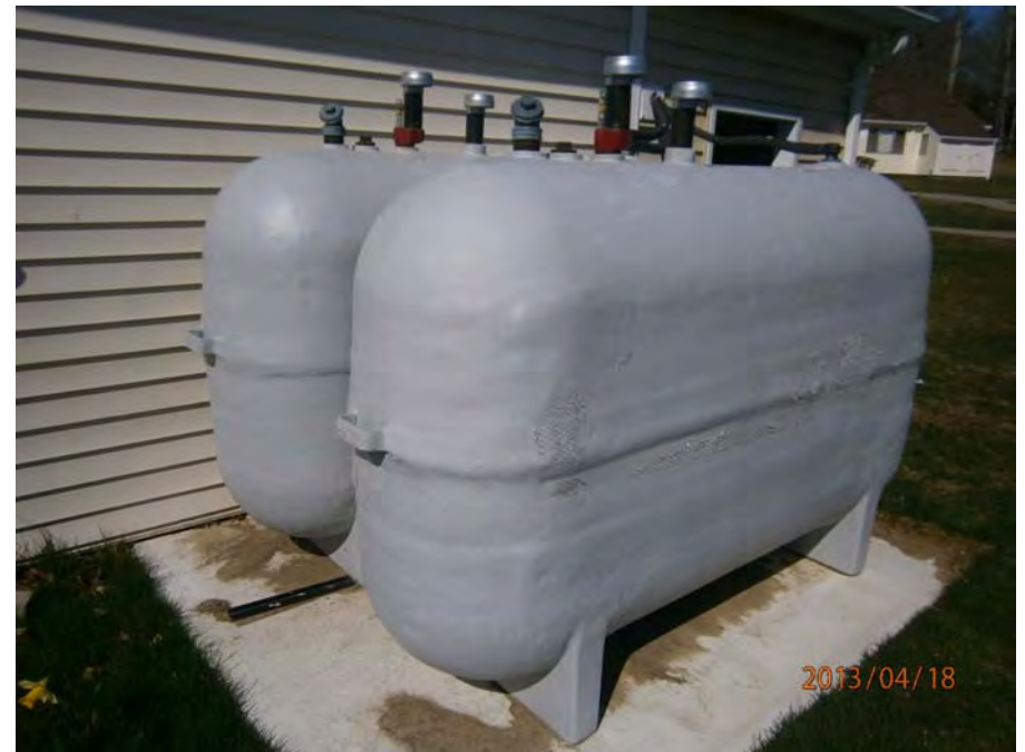
16. Emergency generator fuel tanks
