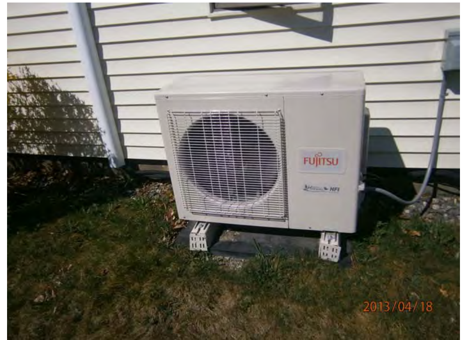
24. Unit split system heat pump
